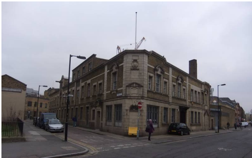
No. 21 Webber Street, the former Maltina Bakery
